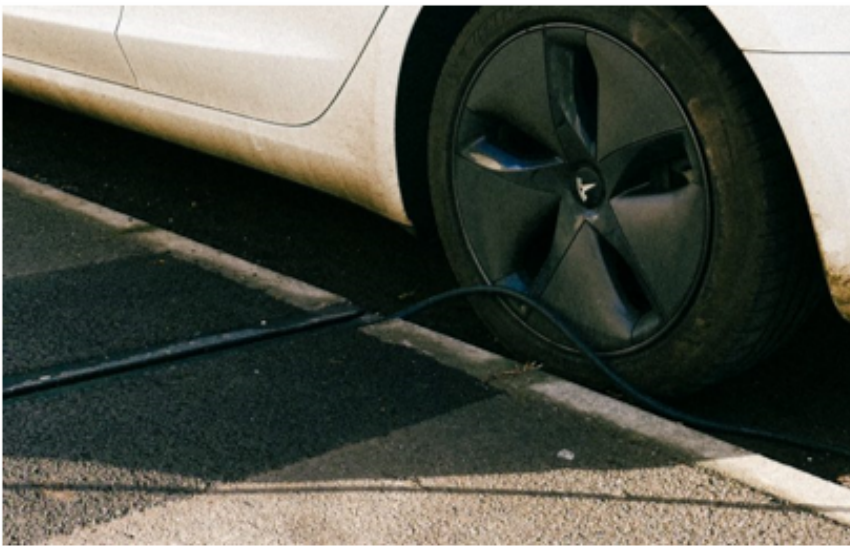
Figure 1 – ODS 'Gul-e' in-pavement cable channels (source: https://gul-e.co.uk/ )
